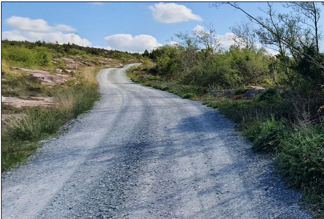
Plate 2-7 Example of unbound (WD4) access track along the grid connection route outside the south of the site (Cal's road).
